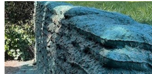
Freshly Hydroseeded Bagwork
