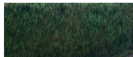
Hydroseeded Bagwork After 6 Months
