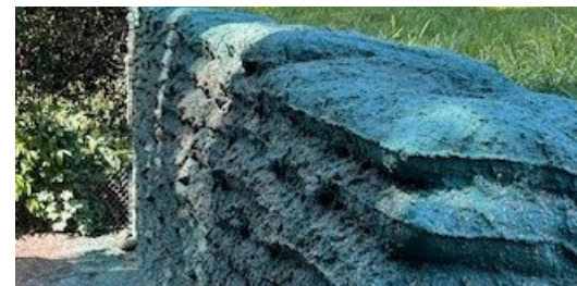
Freshly Hydroseeded Bagwork
